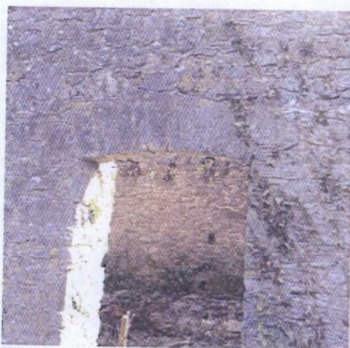
Exterior view of existing opening
