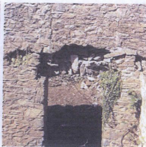
Interior view of existing opening
