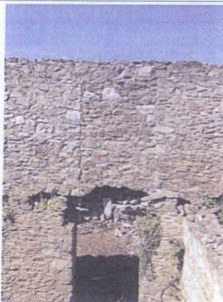
Photo showing historic location of hayloft opening proposed to be reinstated as new window.
