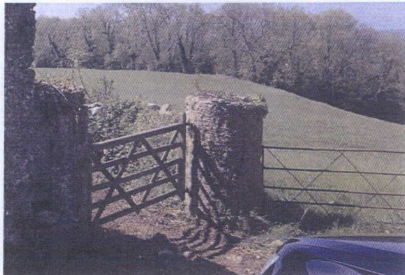
Gateway 3: access from access track within meadow into Linhay enclosure / historic animal pen.
